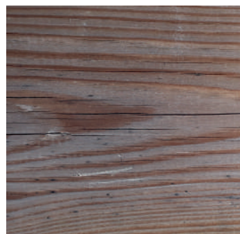
Old wood: after more than 1 year
