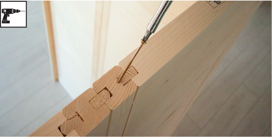
Foret de 3 mm, 8 vis 4 x 70 mm
