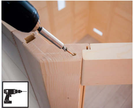
Foret de 3 mm, 1 vis 4 x 70 mm
