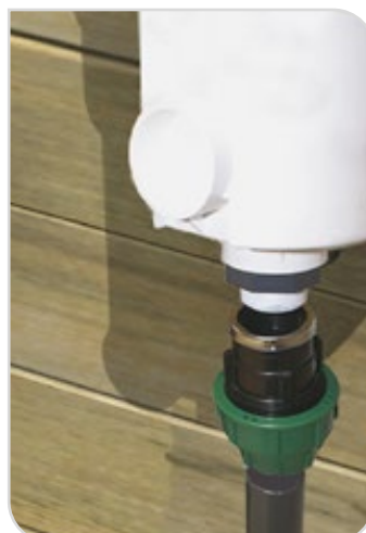
Figure 44 – Raccord du skimmer
